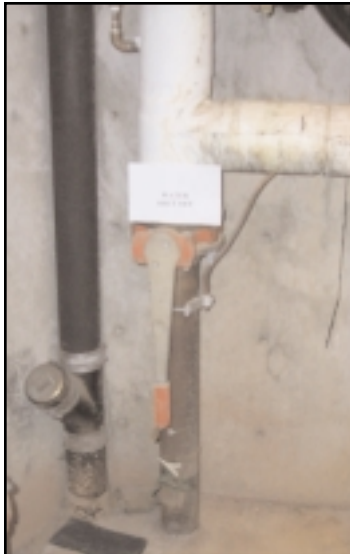
1-4 Main Water Valve
