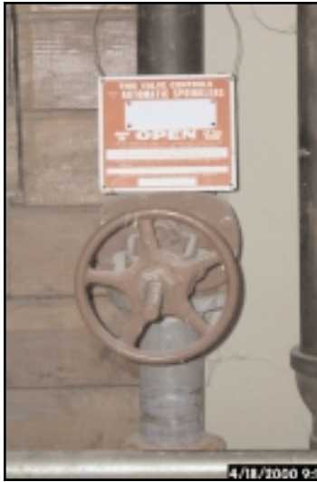
5-1 Fire Sprinkler Main Valve
