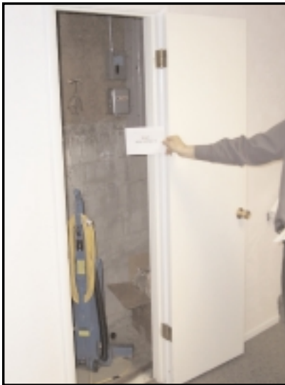
14-3 Main Breaker Panel
