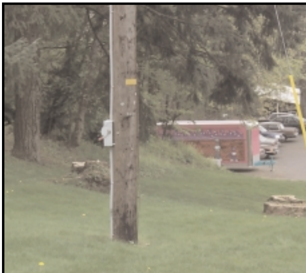
12-1 Disconnect for Auxilliary Pump
