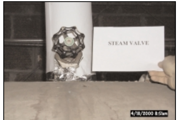
8-5 Bldg. "8" Steam Valve
