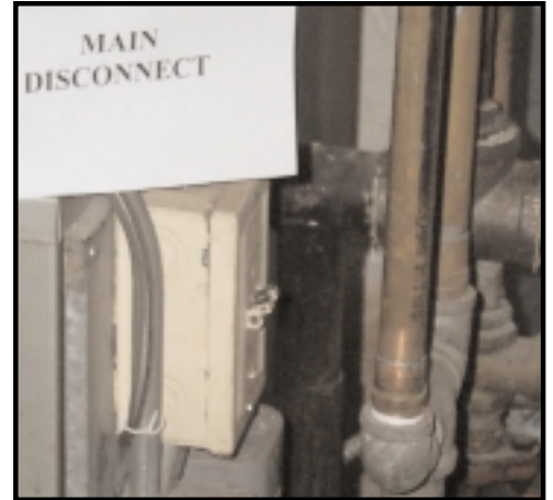
14-2 Boiler Disconnect
