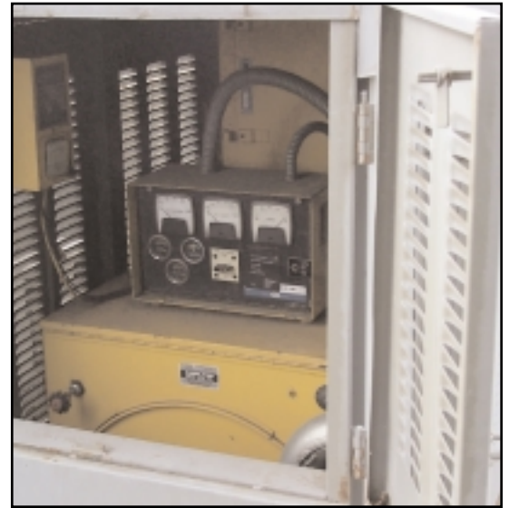
4/3 Emergency Generator Control Panel
