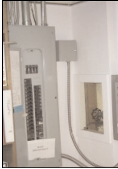
13-2 Main Electric Panel
