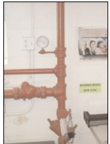
8-7 Fire Sprinkler Valve in Press Graphics Area
