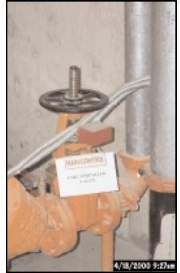
1-3 Main Fire Sprinkler Valve
