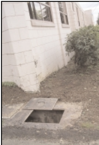
11-1 Steam Valve Pit
