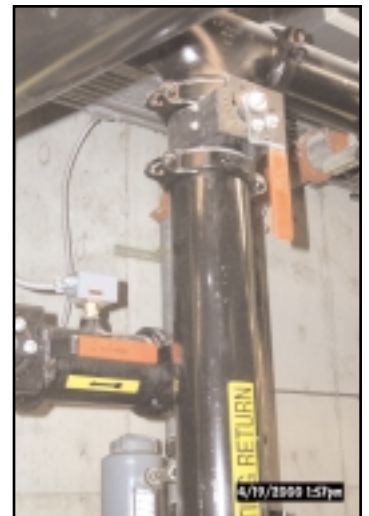
1-8 HVAC - Water Loop Valve
