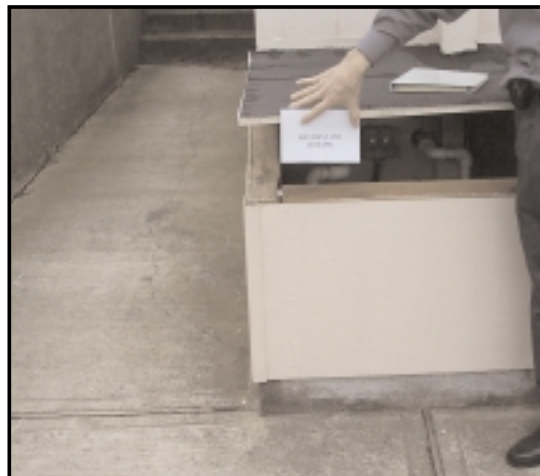
13-6 Steam Condense Return Pump
