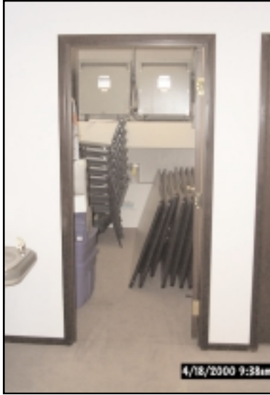
2-1 Upstairs Electrical Closet
