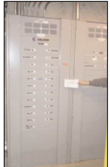
1-6 Main HVAC Panel
