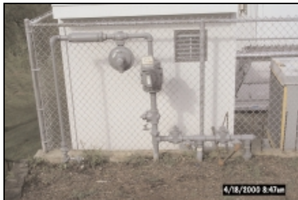
4-4 Gas Valve for Bldgs. 0,1, & 8
