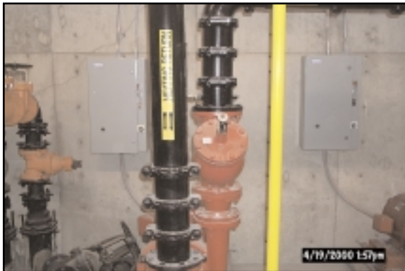
1-7 HVAC - Pump Switches
