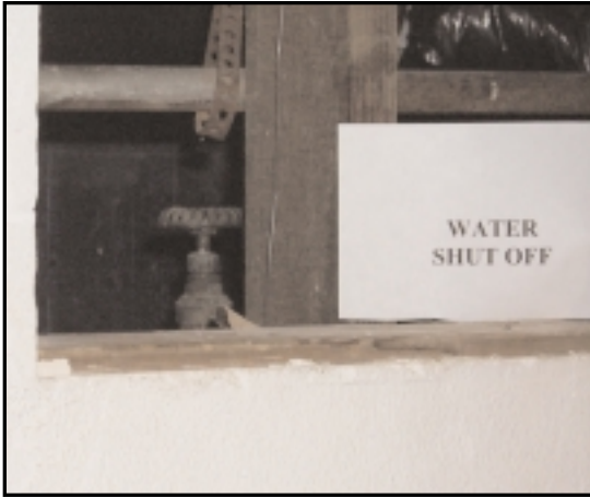
14-1 Main Water Valve
