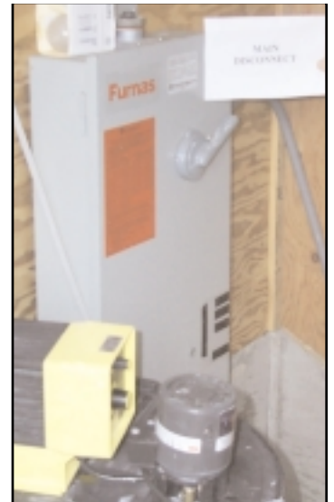
7-2 Main Disconnct for Well Head
