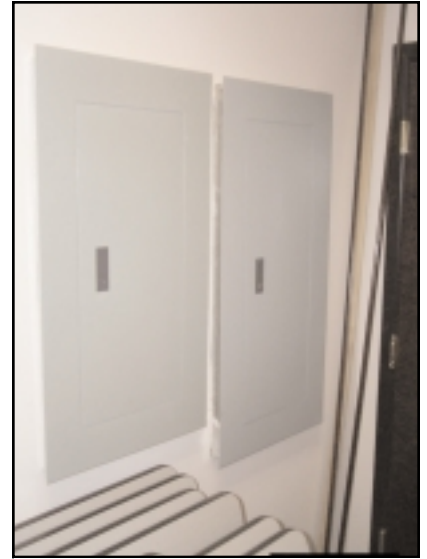
2-2 Upstairs Electrical Panel
