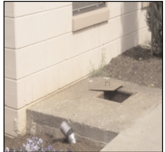
9-1 & 10-1 Steam Valve Pump
