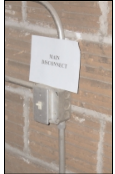
8-3 Boiler Control Switch
