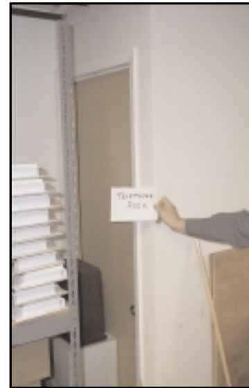
13-5 Telephone Panel Room
