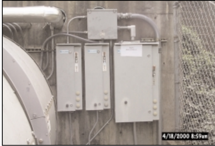
4-1 Cooling Tower Disconnects
