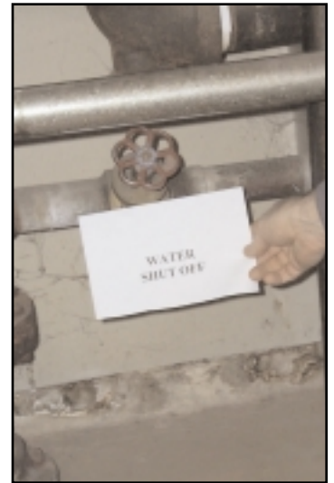
5-2 Main Water Valve
