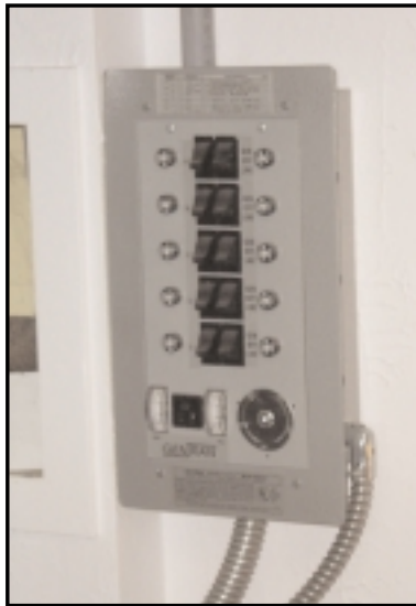
13-4 Emergency Power Panel
