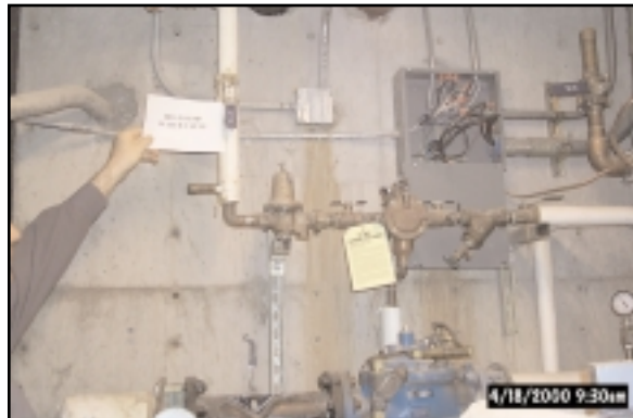
1-5 HVAC - Water Loop Valve
