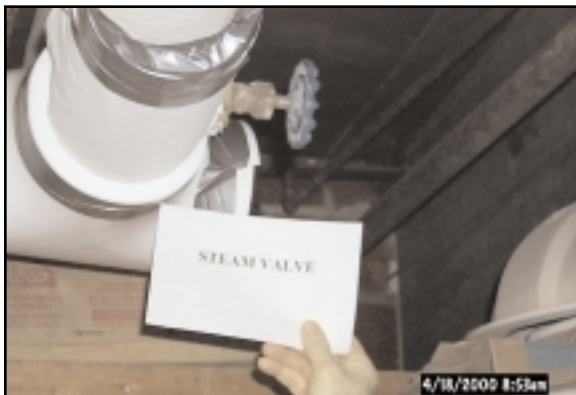
8-6 Bldg. "1" Steam Valve
