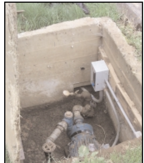
12-2 City Water Auxiliary Pump
